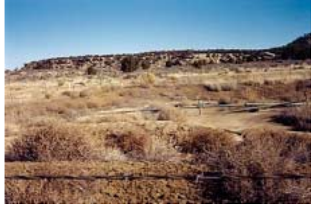
Photo A-14: An unreclaimed open pit used for storing liquid. The fences around them are often disturbed and open to intrusion.
