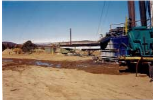
Photo A-10: Leaks from equipment at a well site.
