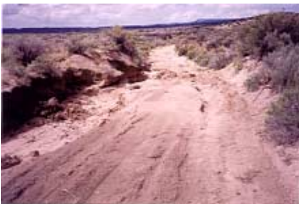
Photo A-5: Old pipeline corridor not re-seeded and experiencing erosion.
