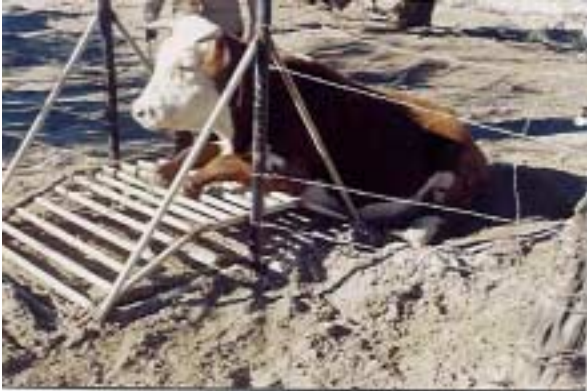
Photo A-1: A Hereford Trapped in a Bicycle Trail Cattle Guard.
