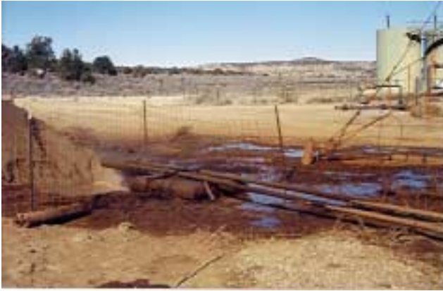
Photo A-13: An active 'open pit' for the storage of liquid waste, along with leaks on the ground.
